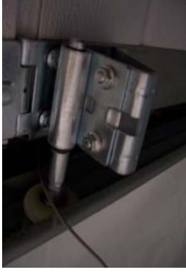
Outer Hinge with roller bearing plate and cable .
